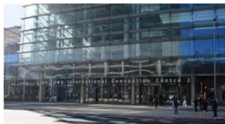
Cape Town International Convention Centre 2, which was officially opened in January 2018 in Cape Town, South Africa. PHOTO: MATHIAS RINGA
